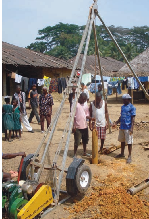
Drilling for Water, Pujehun
